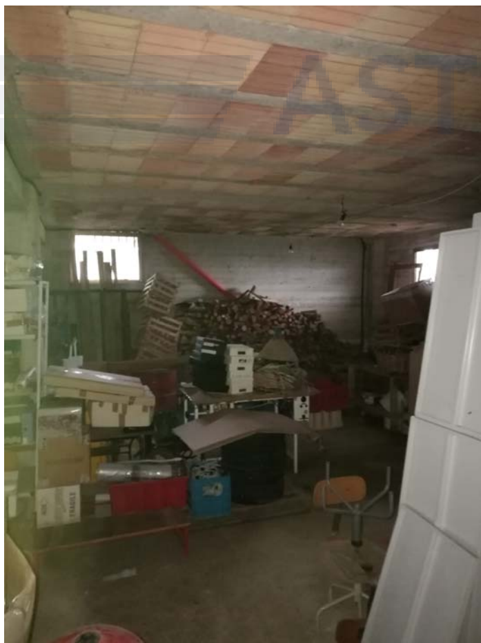
- Garage piano seminterrato
